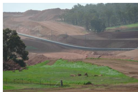
BHP Bauxite Conveyor System, Boddington (S)
