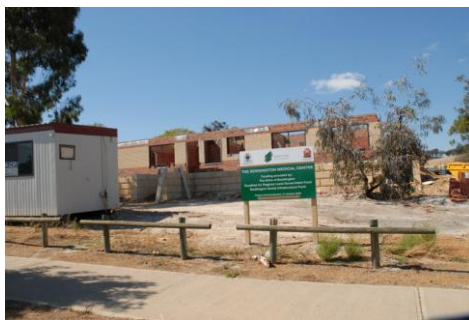
Boddington Medical Centre under Construction
