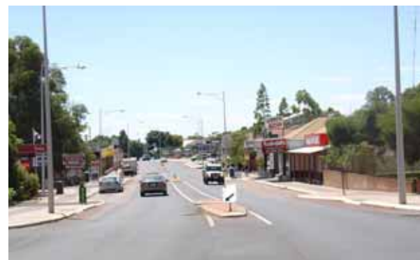
Finishing touches are being applied to Main Street, Waroona
